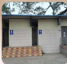
RAILWAY STATION TOILETS
